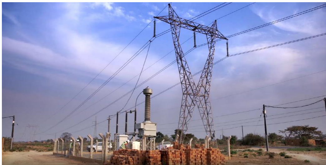
Figure 2. SPT compared to conventional substation.
